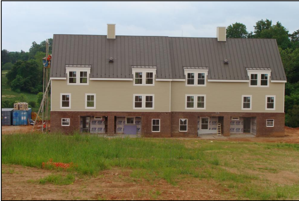
Green Village under construction, view looking from the north side, 5-14-09.
