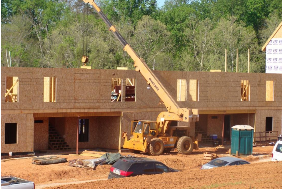
Framing and foundation for east section of student housing, 4-28-09.
